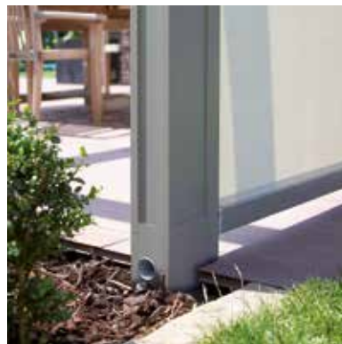
Integrated water drainage
